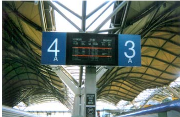
Location of Photograph: Southern Cross Train Station-Spencer Street- Melbourne
